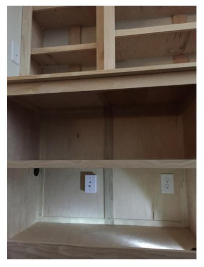
Added ¾ inch plywood at back on left (to fix electrics to). Added ¼ inch plywood at back to right as cheaper and didn't need to fix electrics to it. In the photo above you can see I made the back panel removable incase I ever needed to access the electrics.
